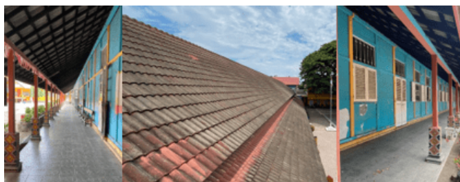
Figure 7 Material used in the building of SMPN 1 Lhokseumawe
