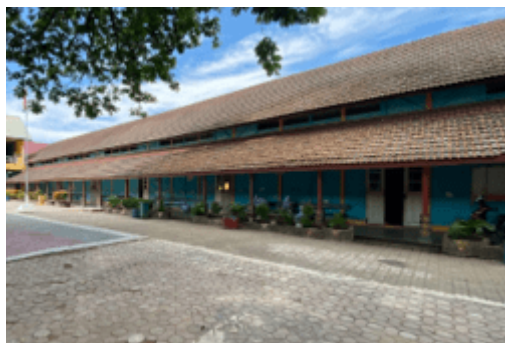
Figure 5 Roof Shape of SMPN 1 Lhokseumawe
