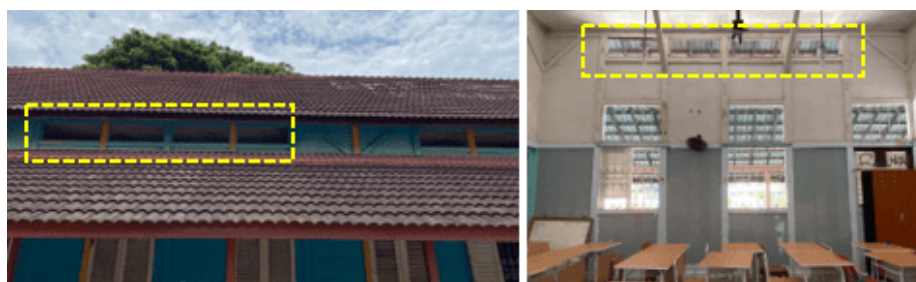
Figure 6 Roof ventilation and clerestory at SMPN 1 Lhokseumawe
