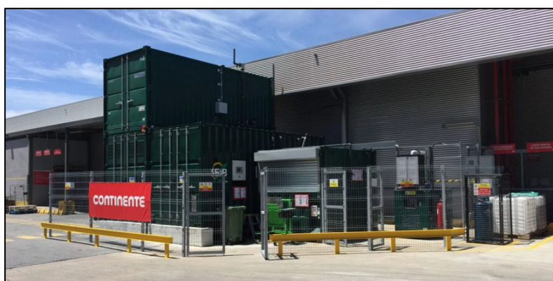
Figure 3 On-site Implementation of the SEaB Energy Flexibuster™ Wet AD System at a Continente Supermarket, Portugal. (Source: SeaB Energy website, 2020)
