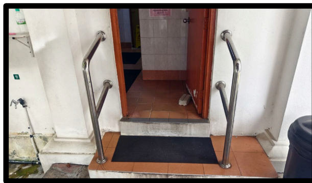
Figure 3 Entrance ramp with handrails leading to an accessible toilet facility (Source: Author, 2026).
