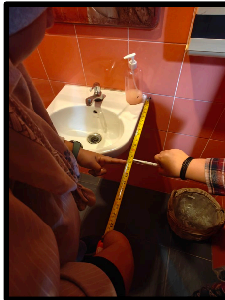
Figure 4 Restricted wash basin clearance within an accessible toilet (Source: Author ,2026).
