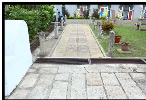
Figure 5 Raised threshold interrupting accessible external pedestrian route (Source: Author, 2026).
