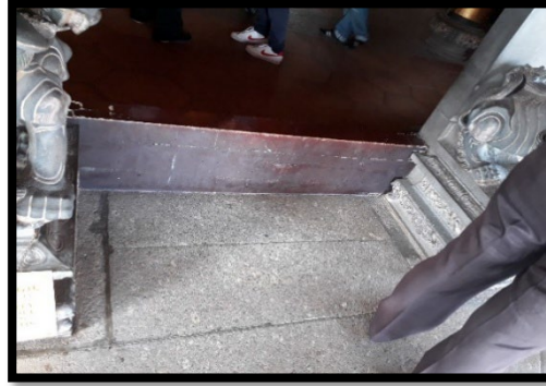
Figure 1 The high sill that prevented the person with disabilities to get to the other side of the building. (Source: Author, 2026)
