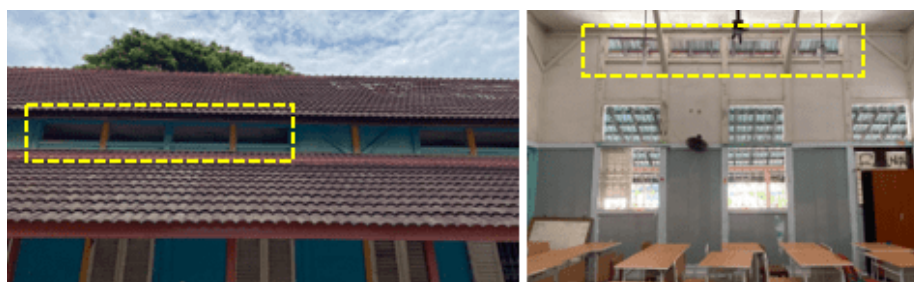
Figure 6 Roof ventilation and clerestory at SMPN 1 Lhokseumawe
