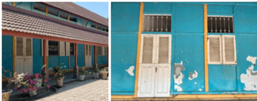
Figure 4 Doors and windows in SMPN 1 Lhokseumawe
